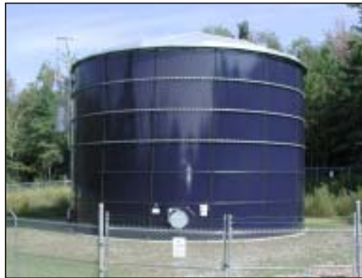
The fence surrounding this storage tank was built after 9/11/2001 to tighten security at one of Vermont's community water systems.
