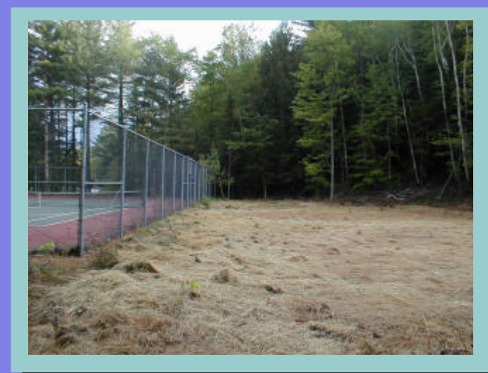
Dispersal System Behind Tennis Courts
