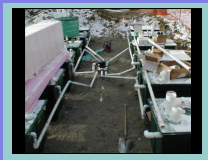
Textile Filter Boxes and Piping Before Covering
