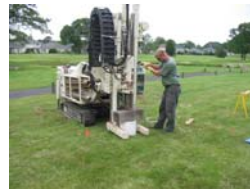
2. Installing the lysimeters.
