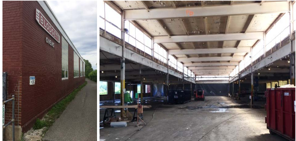
Left: East side of the former Blodgett Ovens factory. Right: Building's manufacturing space undergoing redevelopment.
