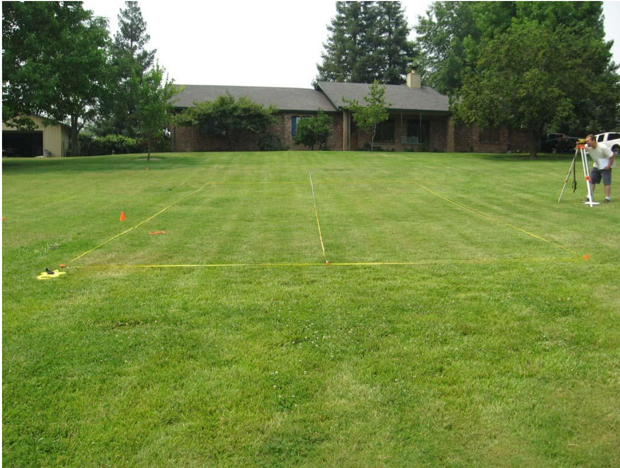
Surveying and laying out plot OIG
