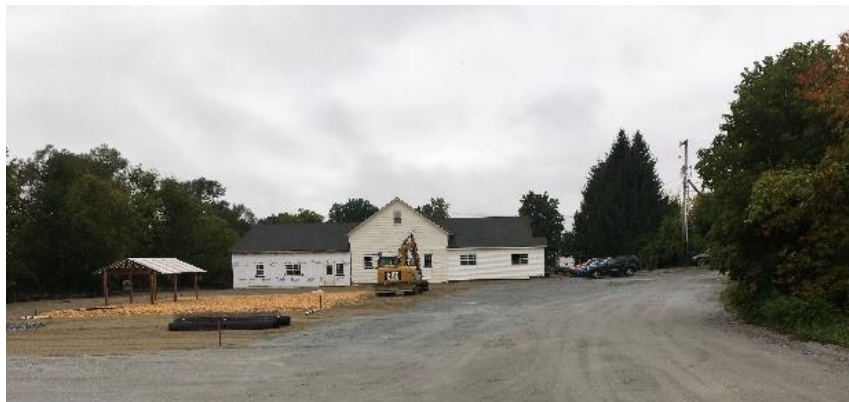
Engineered barriers installed site-wide
