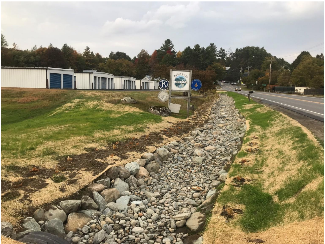
Channel restoration practices near the end of construction, September 2020.
