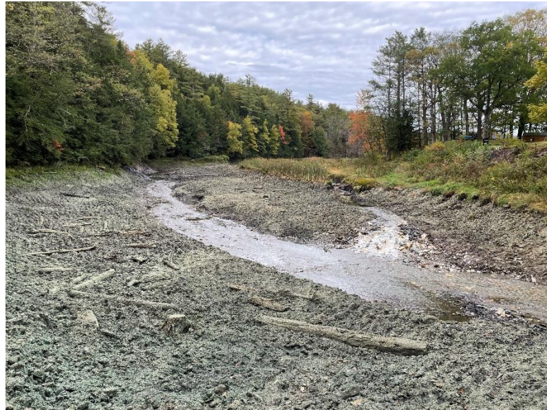
View from the former dam site upstream along the restored channel of North Breton Brook, Castleton, Vermont.
