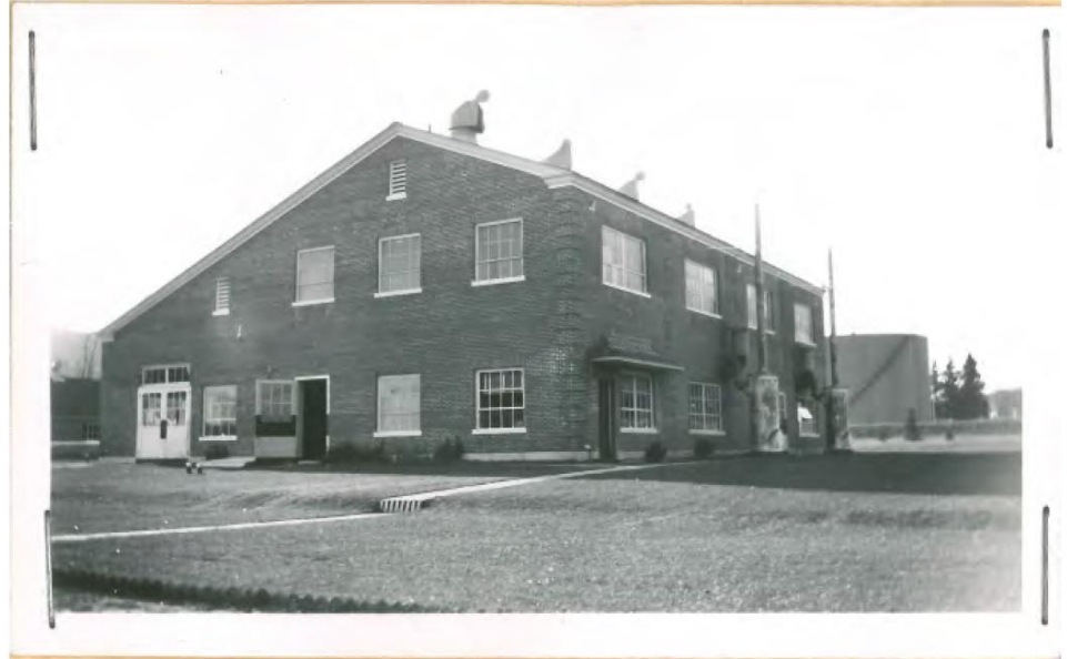
Pump house exterior in 1952. Photo from Terracon Report, 2014
