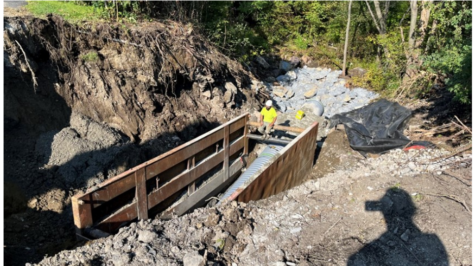
Installation of the new outfall and energy dissipating stone step pools on September 14, 2022.
