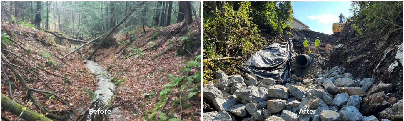
Left: Existing condition in the lower reach of Deer Brook gully, seen in November 2017. Gray-colored water in the channel is due to fine sediment transport during a moderate rain event. Right: Construction of new outfall and energy dissipating stone step pools in September, 2022
