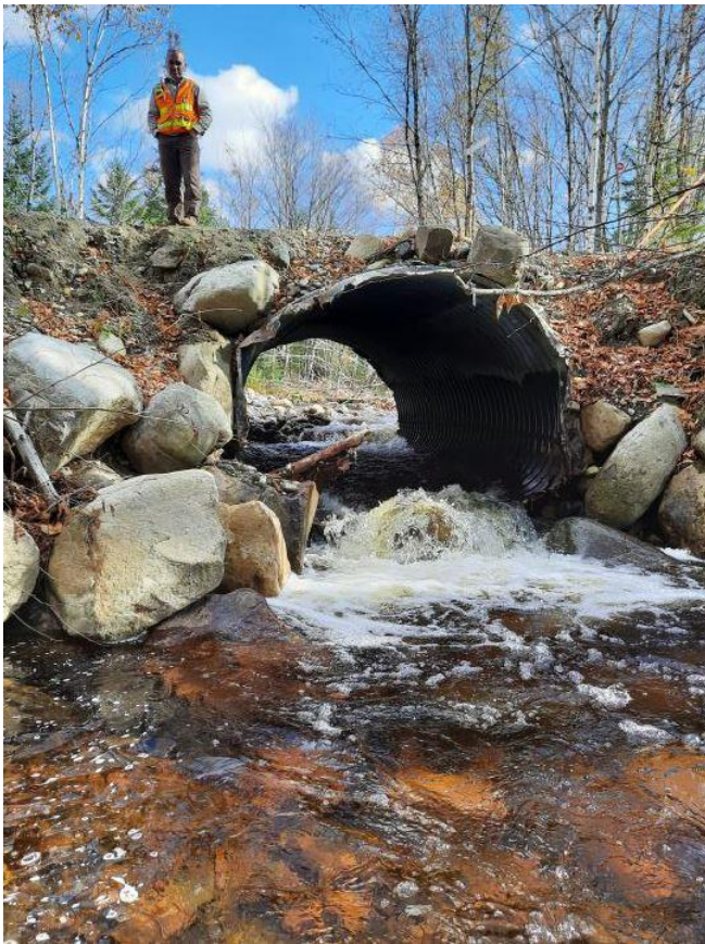
Left: Downstream channel showing aquatic organism passage barrier at Clay Brook in Success, NH. Right: Upstream channel showing headwall and bank degradation at South Branch Sterns Brook
