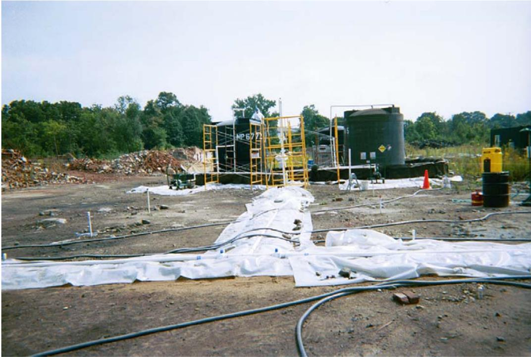
*Figure 24. Permanganate Mixing Tanks and Distribution Manifold.*
