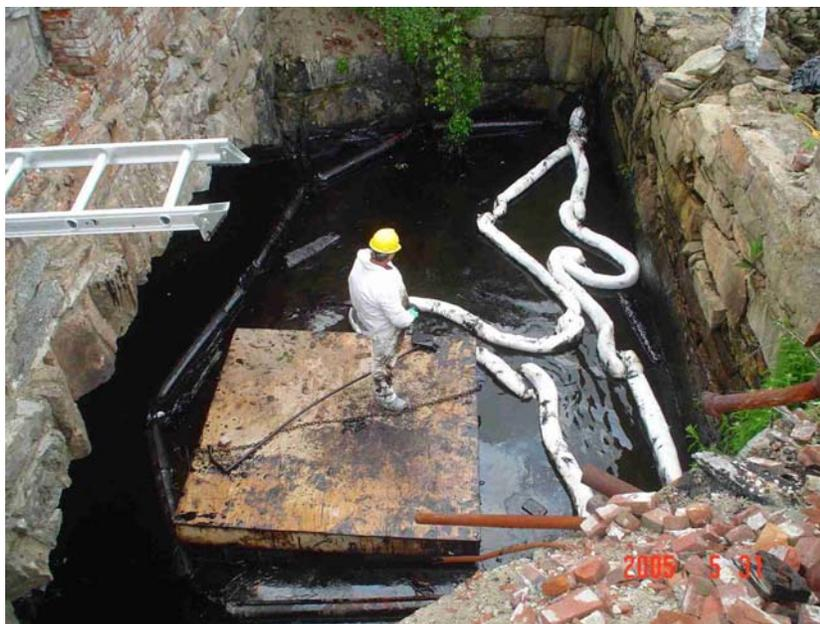
*Figure 34.* Oil absorbent boom change out in canal near tailraces
