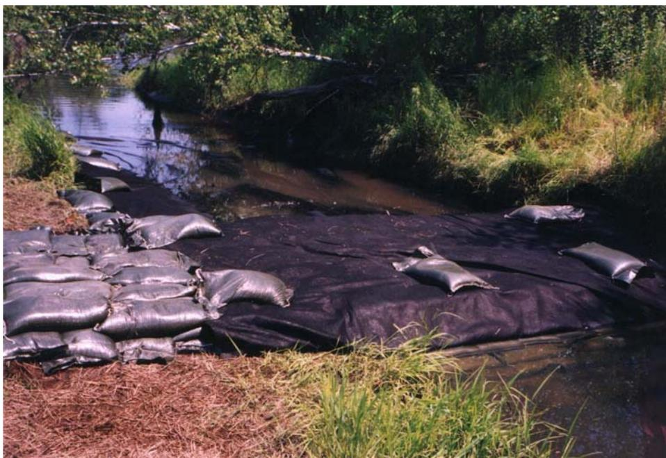
*Figure 15.* Sand bag dam installed in June 2002.
