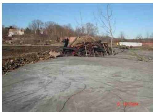
*Figure 31 (left).* Application of flowable fill to encapsulate debris. *Figure 32 (right).* Flowable fill after setting and curing.
