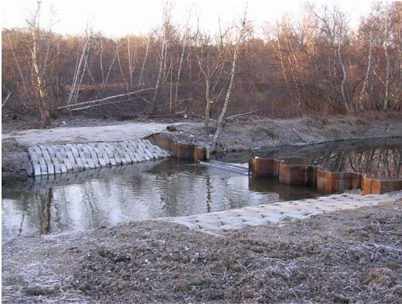
Figure 16. Sheet-piling dam installed in December 2003.
