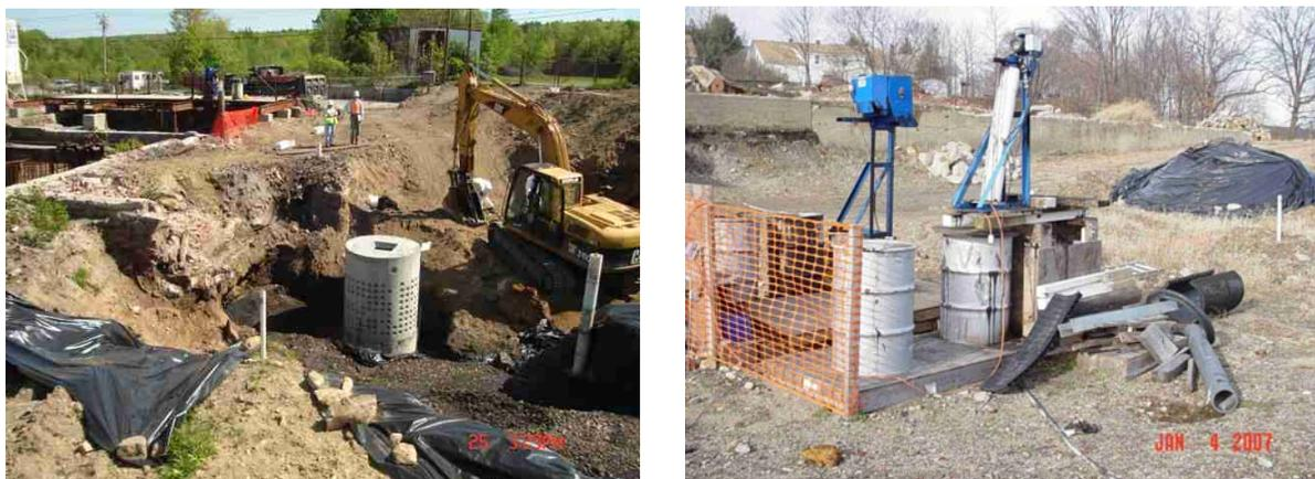
*Figure 39(left).* Installation of one of two recovery wells using perforated leaching basin sections.; *Figure 40(right).* Recovery wells fitted with belt skimmers.
