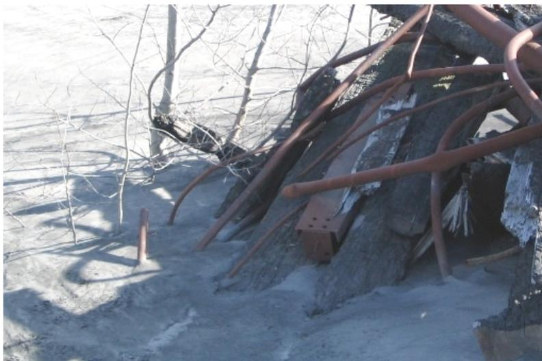
*Figure 30.* Encapsulation of debris with flowable fill.
