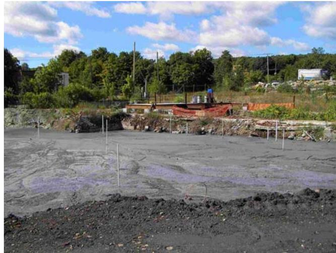
*Figure 33.* Application of flowable fill in front foundation area in conjunction with SVE piping, monitoring wells and injection points.
