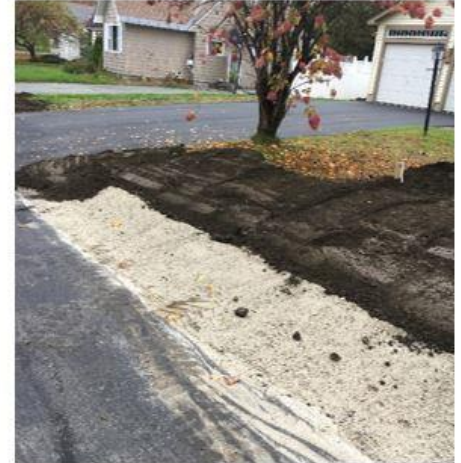
Construction of a bioretention swale with an underdrain at the drain outlet designed to allow water that is unable to infiltrate to flow to the stormwater collection system (left) and photo of a bioswale following construction (right).
