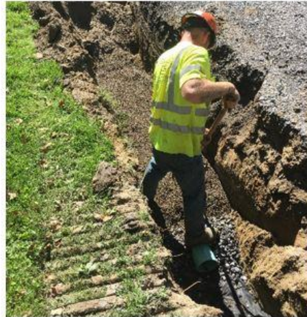
Construction of a bioretention swale with an underdrain at the drain outlet designed to allow water that is unable to infiltrate to flow to the stormwater collection system (left) and photo of a bioswale following construction (right).
