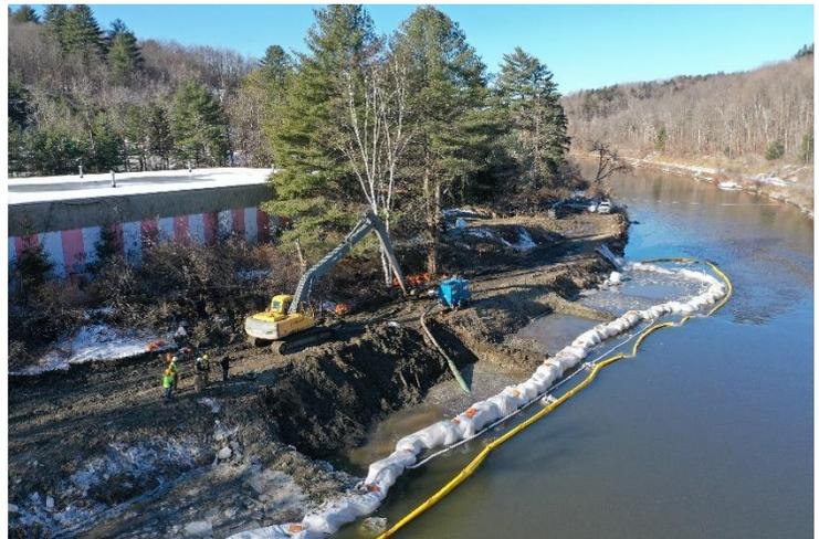
*Top: Tar released to the ground surface on the bank of the Winooski River. Bottom: Excavation crews employ a coffer dam in the Winooski River while removing coal tar contaminated soils. Photos by Stone Environmental*
