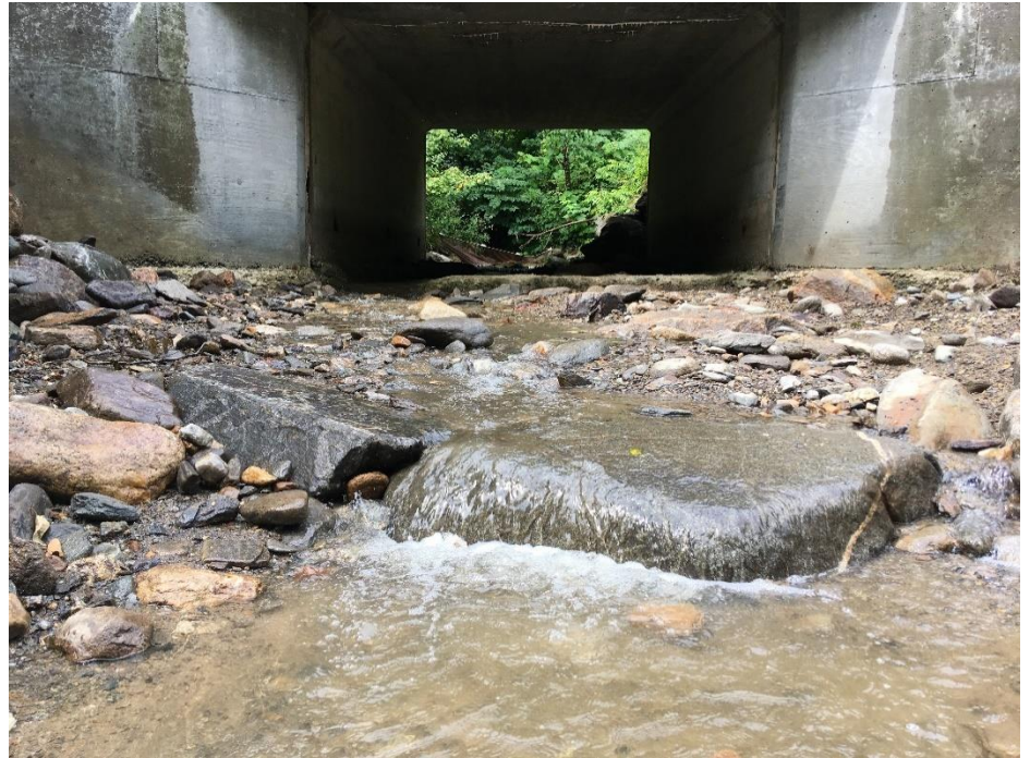
The grade control structure, made of boulders, seen downstream of the NHDOT culvert.
