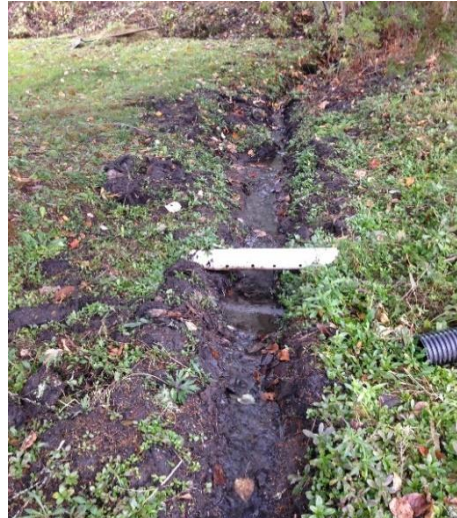
Photographs from Montpelier's Chestnut Hill neighborhood display a lack of adequate drainage and significant sediment load that resulted in flooding.
