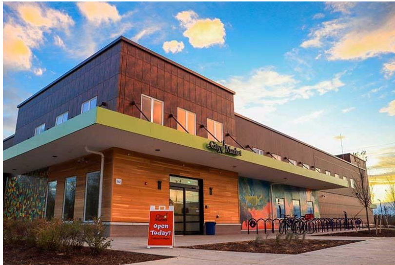
Photo of the new coop following remedial implementation and construction. Source: City Market
