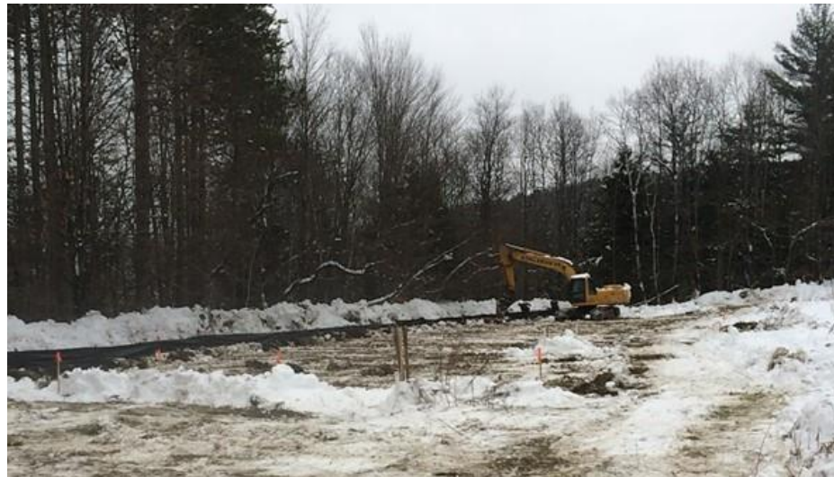
The pilot community wastewater treatment system's leachfield under construction in Irasville
