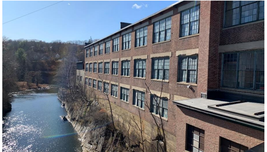
Comtu Falls three story brick building located in downtown Springfield, Vermont.
